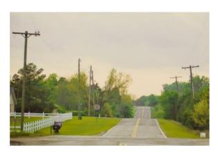
The operator of a vehicle traveling at 40 miles per hour along a rural roadway must be able to observe the roadway beyond two (2) utility poles, to see and safely for a hazard.
